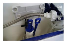
Instal Toilet Water Saver. Twist and lift blue mechanism piece out of the way and insert and hang Toilet Water Saver inside overflow tube.
